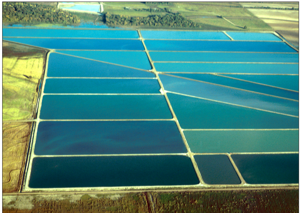
Figure 1. Aerial view of levee ponds.
