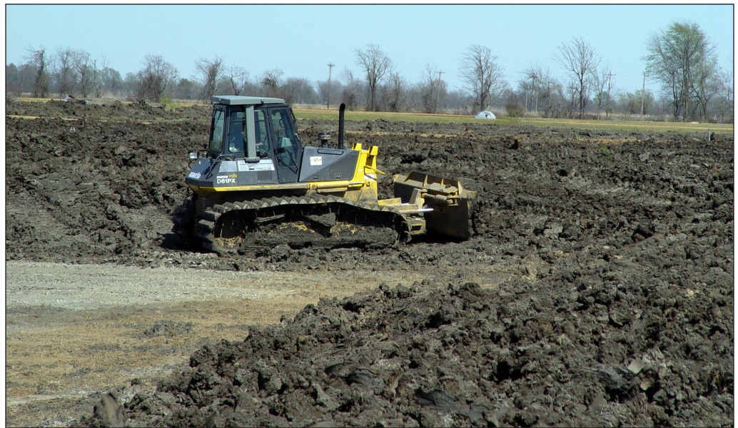
Figure 3. Bulldozer constructing levees.
